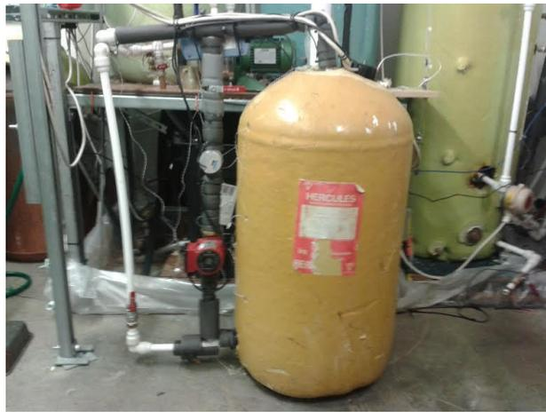
**Figure 3-15 Photograph of tank from flat a retrofitted with destratification pump**
